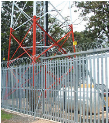
Alan Dick East Africa has used hundreds of Cat® and Olympian™ generator sets to supply power for cell sites.
