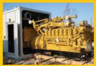
With only four months to transport and construct a complete heat and power facility to support the city of Bogorodskoe, Caterpillar and local dealer Amur Machinery commissioned three G3516B generator sets in arctic grade enclosures with a heat recovery system that delivers 90 percent system efficiency.
