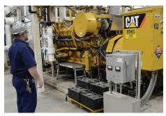
Four Cat® G3516B gas generator sets produce 2.4 MW of power, enough to provide 92% of the power required to run the wastewater plant portion of the facility.
