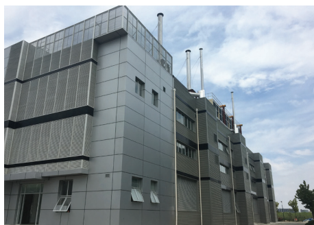
The Shanghai Tencent Cloud Data Center (TCDC) is one of the most advanced service platforms for cloud computing and cloud storage infrastructures in the Asia-Pacific region.
