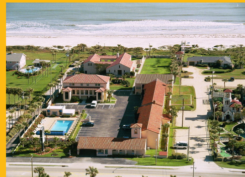
An aerial shot of La Fiesta Ocean Inn shows the property prior to Hurricane Matthew.
