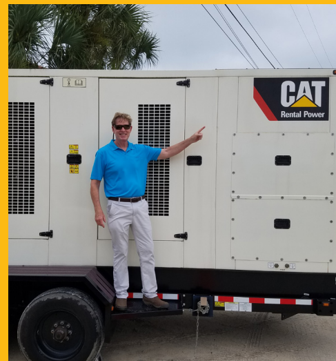
Rich O'Brien, owner of the La Fiesta Inn, stands with the Cat® XQ400 generator set that supplied power to the 46-room hotel.
