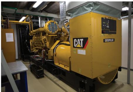
*Together with Cat® dealer Zeppelin Power Systems, DataSpace designed an infrastructure featuring six Cat 3516B diesel generator sets to provide reliable backup power.*
