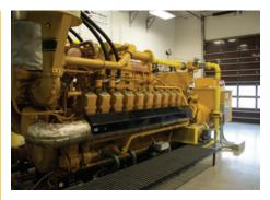
Granger pumps 10,000 standard cubic feet of methane per minute to four Cat® G3520C generator sets to convert the gas to a reliable energy source.
