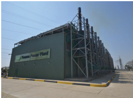
The newly upgraded Ywama Power Plant in Yangon, Myanmar, delivers an additional 50 MW of power to the city, representing four percent of country's entire power supply.
