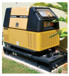
One of the most appealing features for residential settings is the quiet operation of Olympian™ generator sets, enabled by sound absorbent materials, an improved exhaust system and better managed airflow.
