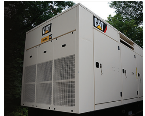
Monticello uses a 500 kW Cat® C15 diesel generator set equipped with a sound attenuated, weather-protected enclosure to minimize noise.
