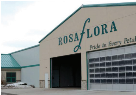
Rosa Flora improves energy efficiency with a number of conservation strategies including a new combined heat and power (CHP) system for its 40-acre greenhouse facility.
