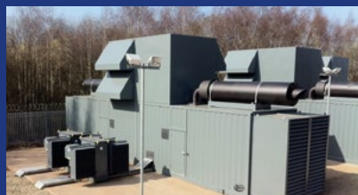
Pictured: Twin pack sound attenuated enclosures for 2 X AJ1870 Perkins powered 4012-46TAG3A engines.
