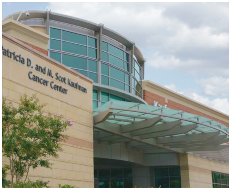
UM UCMC utilized combined heat and power (CHP) to improve system reliability.
