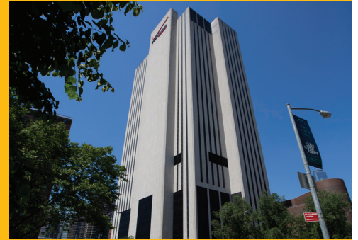
Intergate.Manhattan is the tallest high-rise data center in the world.
