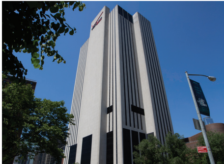
Intergate Manhattan is the tallest high-rise data center in the world.
