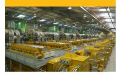
Rubart Station runs on 12 Cat® G20CM34 natural gas-fired RICE units for 110 MW of flexible utility power that meets efficiency and emissions requirements.
