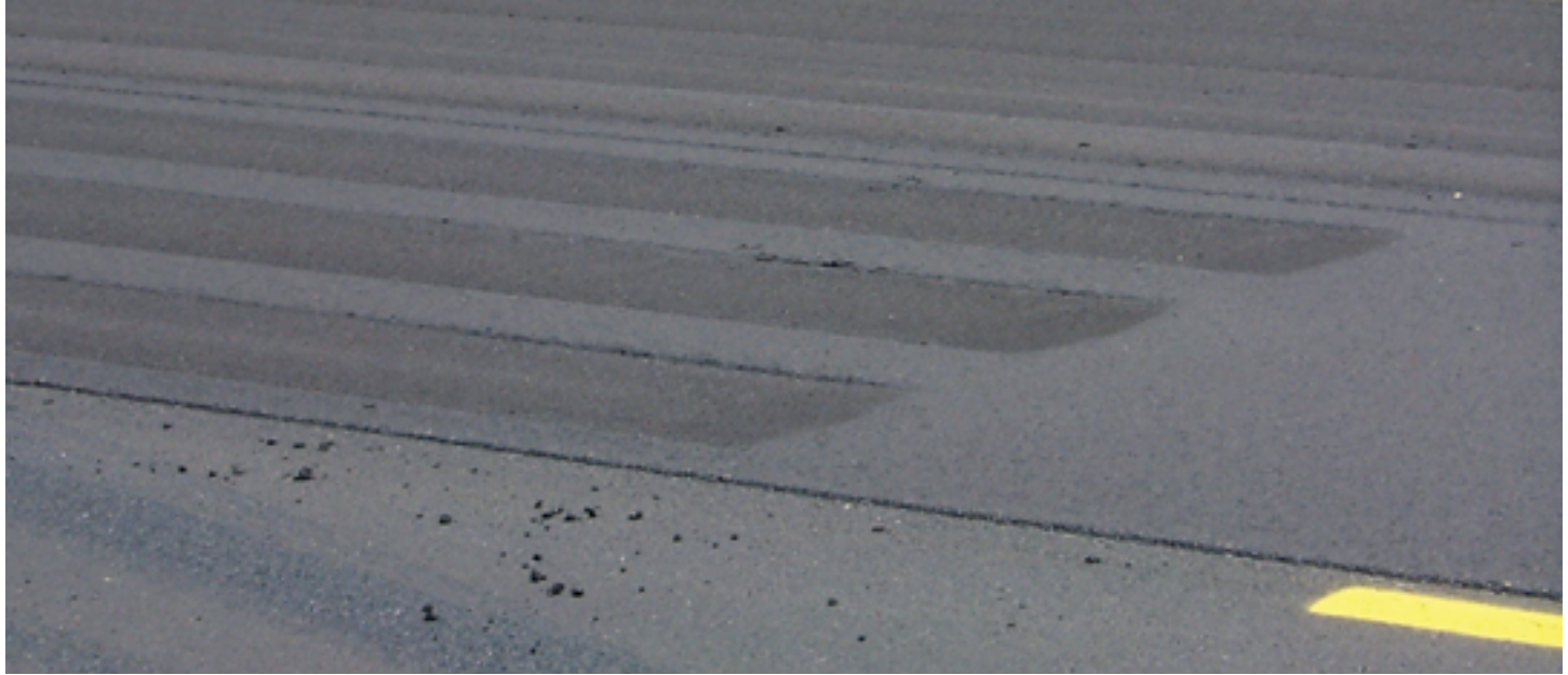
Pneumatic compactors are allowed to stop straight on the mat.
