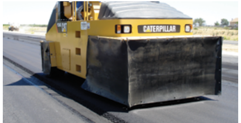
Pneumatic compactors always stay at least 15 cm (6") from unconfined edges.
