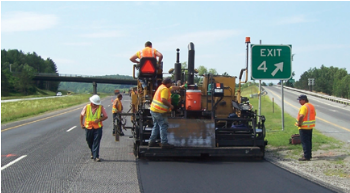
Paving emergency lanes first improves the smoothness of adjacent driving lanes.
