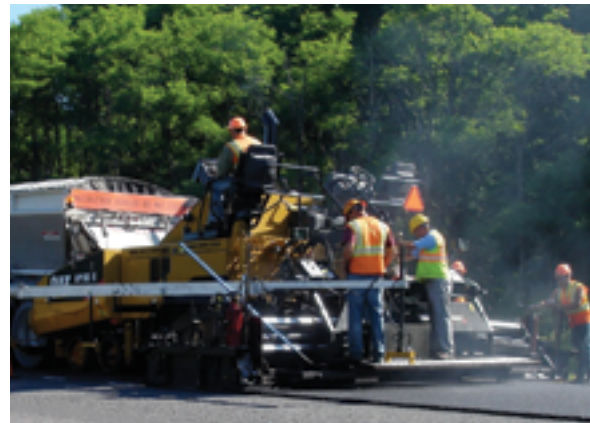
Non-contact skis offer convenience and adequate averaging for surfaces with light to moderate roughness.
