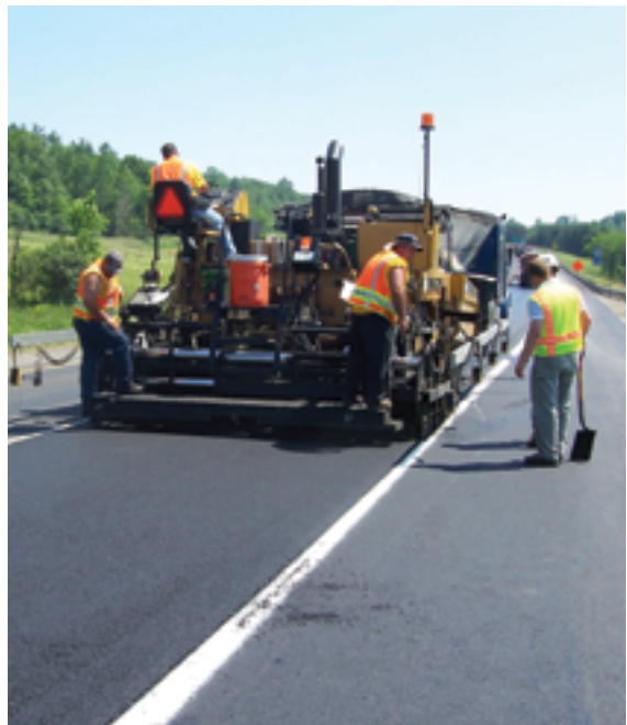
Averaging ski using emergency lane as a grade reference.
