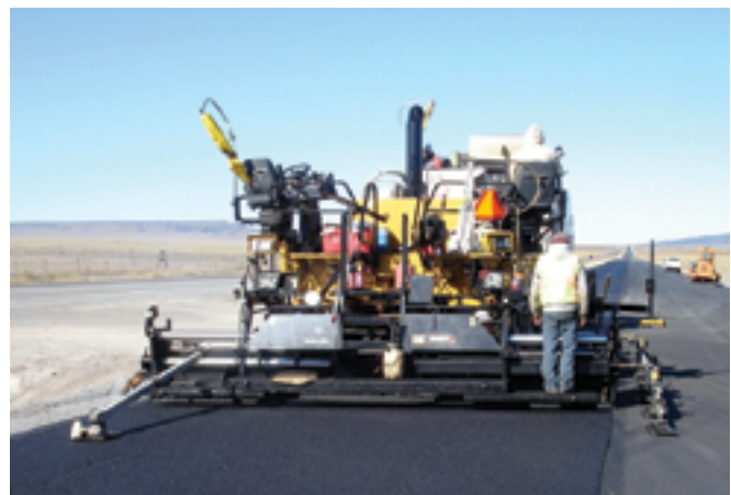
Dual, mechanical averaging skis can produce up to a 60-70 percent improvement in one-pass smoothness.
