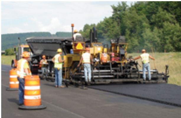
Create a vertical unconfined edge by running the screed end gate in the float position on the grade being paved.
