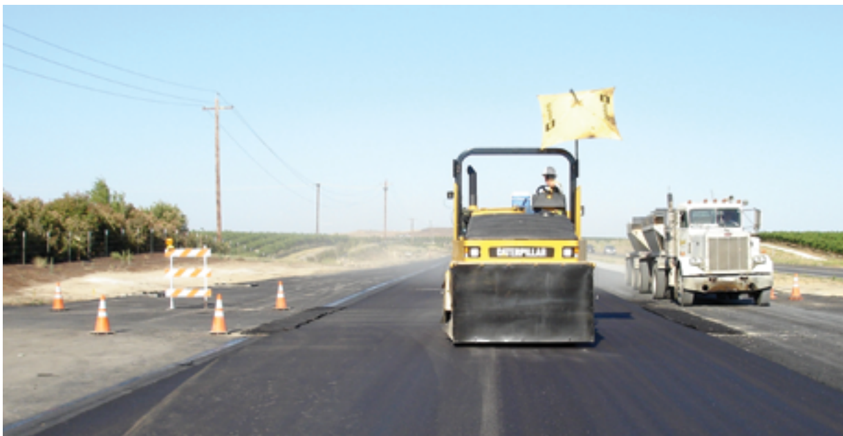
Pneumatic compactor sealing a hot / cold longitudinal joint.
