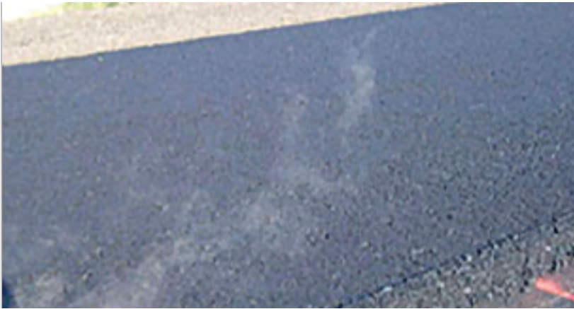
Temperature variation caused by 10-minute paver stop. Screed imprint seen in infrared image is not visible in digital image.
