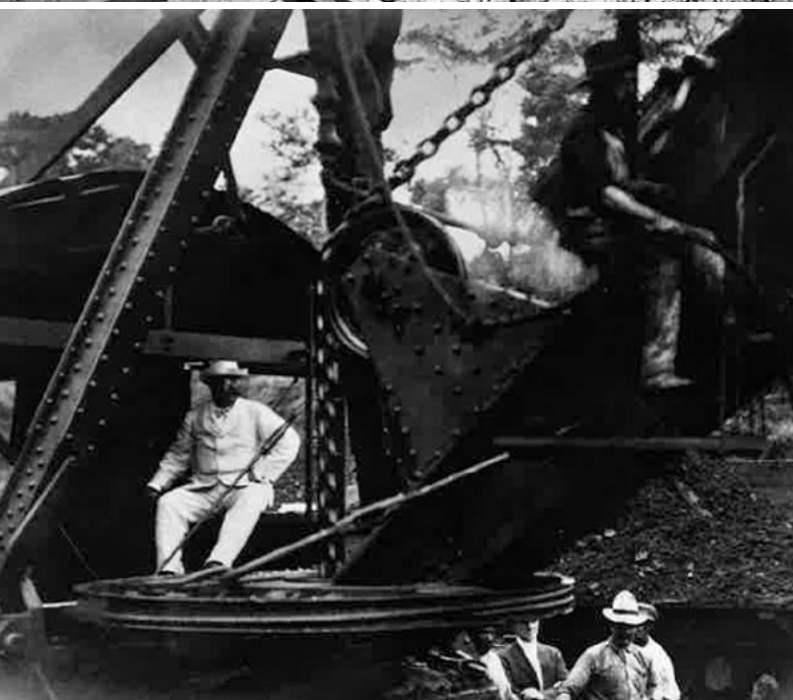
Steam shovels like these — the predecessors of today's Cat® mining shovels — played a major role in public works in the 19th and early 20th centuries, being key to the construction of railroads and the Panama Canal. Many were built on railroad chassis, on which the boiler and engines were mounted. U.S. President Theodore Roosevelt, in far left photo, posed on a steam shovel during his visit to the Panama Canal site in 1906.
