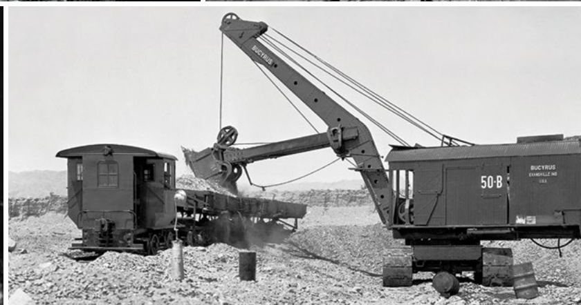
Steam shovels like these — the predecessors of today's Cat® mining shovels — played a major role in public works in the 19th and early 20th centuries, being key to the construction of railroads and the Panama Canal. Many were built on railroad chassis, on which the boiler and engines were mounted. U.S. President Theodore Roosevelt, in far left photo, posed on a steam shovel during his visit to the Panama Canal site in 1906.
