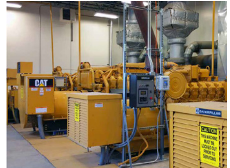
The G3520 is a high-power density 20-cylinder engine offering market leading load acceptance and transient response.
