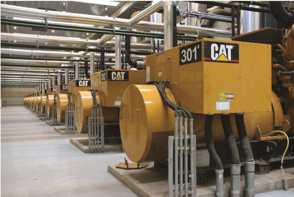
Figure 2: The interior of one of four coal gas power plants that utilize exhaust heat recovery steam generators to power a 3 MW steam turbine.
