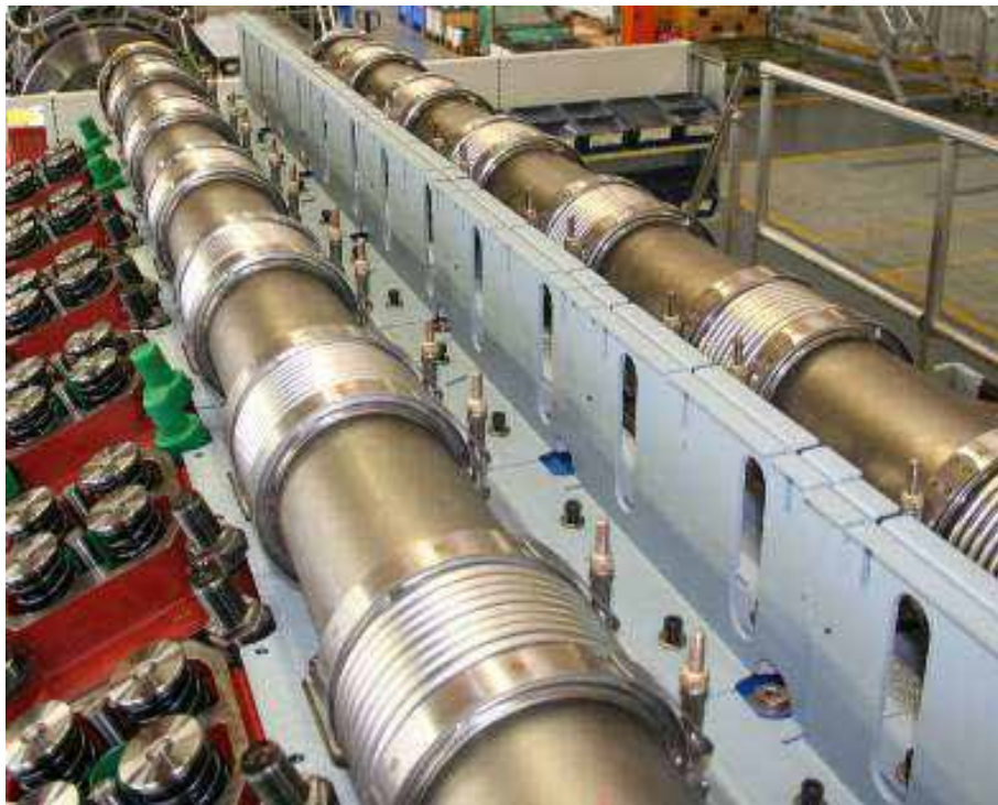
Figure 8: Pulse energy advanced recovery line
