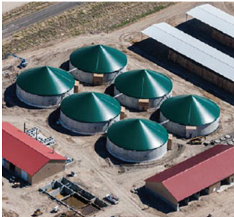
To mitigate odors, Bettencourt Dairies installed six one-million-gallon anaerobic digesters on site to process manure at Rock Creek Dairy.
