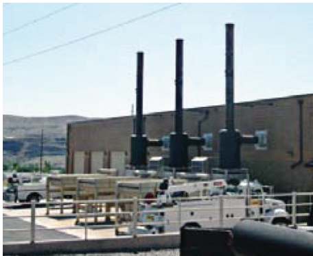
Hurricane City Power Plant
