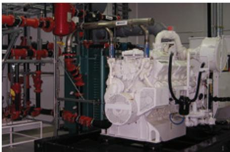
The cogeneration plant provides more than 100 percent of PEPCO's electricity needs and 95 percent of its heating and cooling needs.
