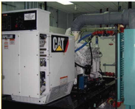
PEPCO selected a Cat® G3412C generator set for its cogeneration plant. The installation is intended to showcase the PEPCO-designed control system, which operates not only the cogeneration plant but also most of PEPCO's headquarters building. The white finish is a custom touch inspired by the typical finish in a ship's control room.
