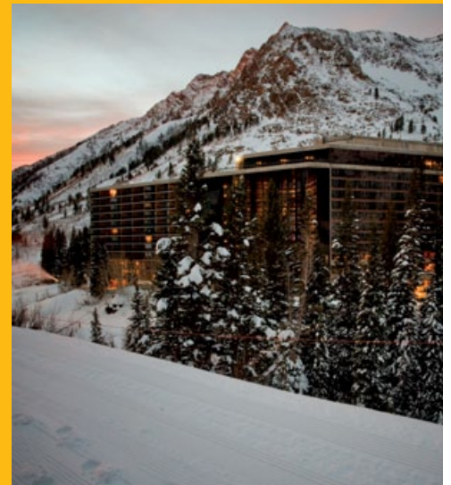
The 562-room Cliff Lodge & Spa at Snowbird uses heat and electricity from a combined heat and power (CHP) solution driven by Cat® gas generator sets.
