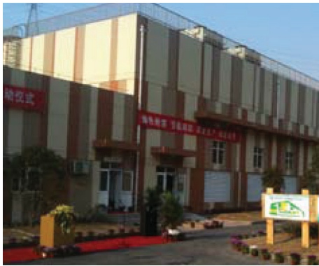
This landfill gas-to-power generation plant in Hangzhou, China, was developed with government tax incentives and has helped increase the capacity of the local power grid.
