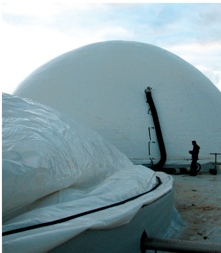
Using two-stage agriculture biodigestion technology, Seacliff transforms vegetable and animal waste into heat, electricity and natural fertilizer.
