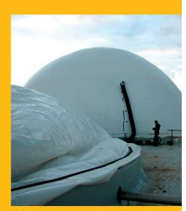
Using two-stage agriculture biodigestion technology, Seacliff transforms vegetable and animal waste into heat, electricity and natural fertilizer.
