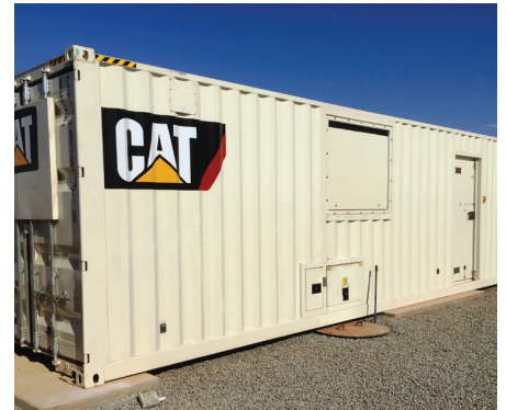
30 Cat® XQ2000 power modules supply 35 MW of power to the Roy Hill Iron Ore Facility.
