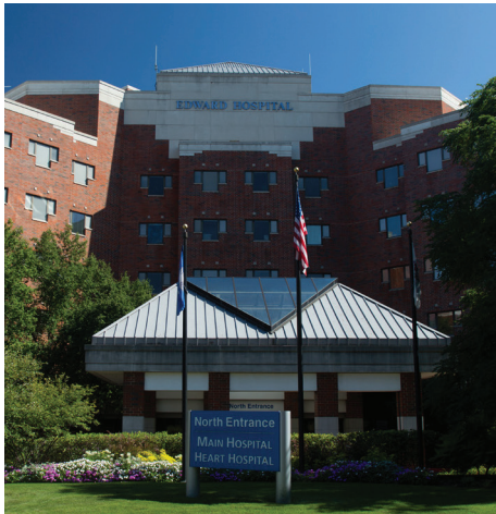
Edward Hospital & Health Services overcame sound and space constraints with a customized standby power solution to better support mission critical needs.
