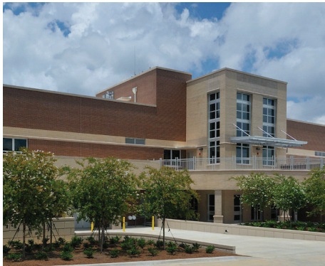
The Leon County Government and the City of Tallahassee combined the 911 dispatch and emergency response functions from both locations at a new 90,000-square-foot Public Safety Complex to improve emergency response time.
