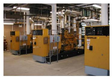
Three Cat® G3406 generator sets provide power for the Westmount complex along with heat for its boilers and laundry system. Operated by Siemens Building Technologies, the plant can be managed remotely to adjust for changing conditions.
