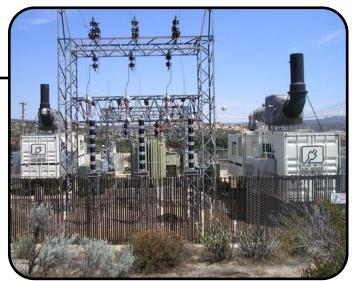
These two Cat 3516B diesel power modules supplied by Hawthorne Power Systems provided power to a small California community during daylight hours while electric utility crews installed new transmission lines for a 50 MW wind farm.
