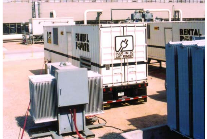
The job required three 4160-volt transformers, three 4160-volt disconnect switches and more than three-quarters of a mile of cable.
