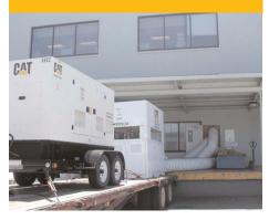
A 30-ton, 10,000 cfm chiller from NC Power was connected to a 100 kW XQ100 sound-attenuated generator on the loading dock of the Fred Hutchinson Cancer Research Center in July, 2006. It took NC Power just four hours to gather the equipment, transport it, set it up and get the system running when the Center's cooling system failed.
