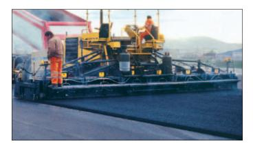
**Screed choices.** The AP755 is available with the AS3251 screed and the AS4251 screed both available with variable frequency tamper and vibrators and with LPG and electric heating system. Also available are the RB 5700 hydraulic LPG screed and the RMB mechanical LPG screeds.
