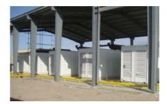
or mains supply of power. The 4012-46TWG2A's power containerised 1250 kVA diesel generators which provide heat, light and hot water for the base and light for an operational runway. Read the full case study **here**
