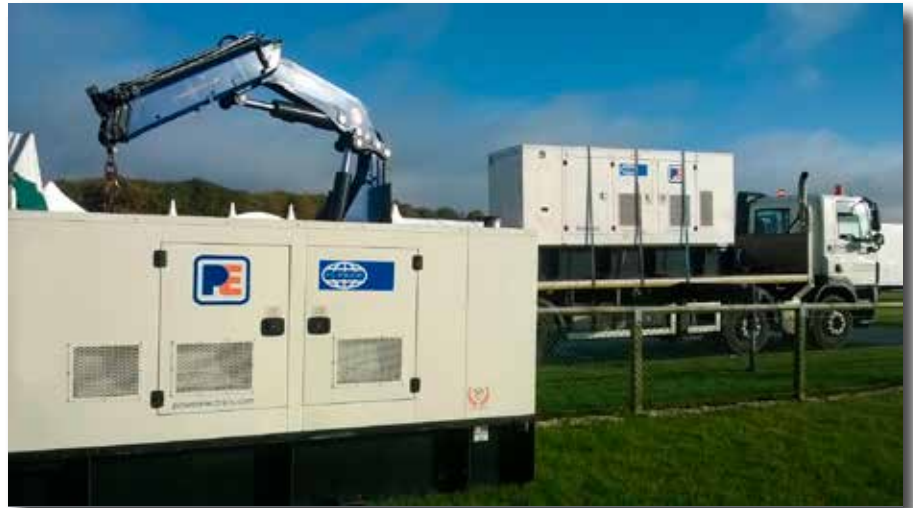
30 rental generator sets ranging from 60 – 500 kVA providing power for a large exhibition at Newbury Showground, UK.
