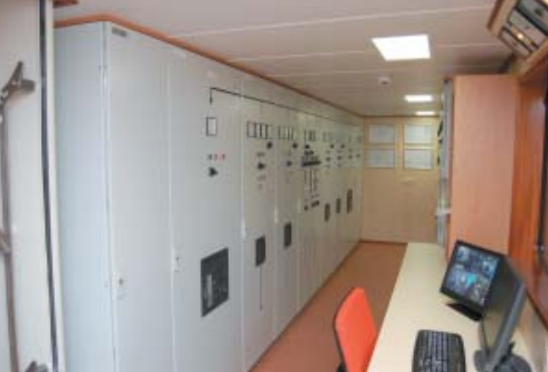
The electrical installation was done by GTI Suez
