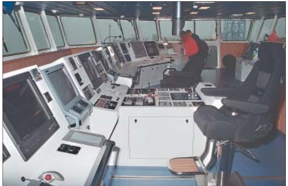
Eekels Elektrotechnik supplied the control consoles for navigational aids and communication systems
