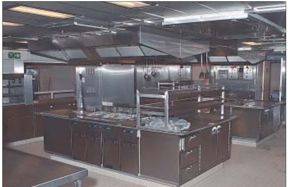
The complete galley system has been designed by Imtech Marine & Offshore
