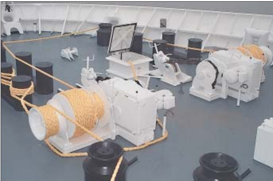
Deck equipment includes SEC anchor windlasses and mooring equipment
