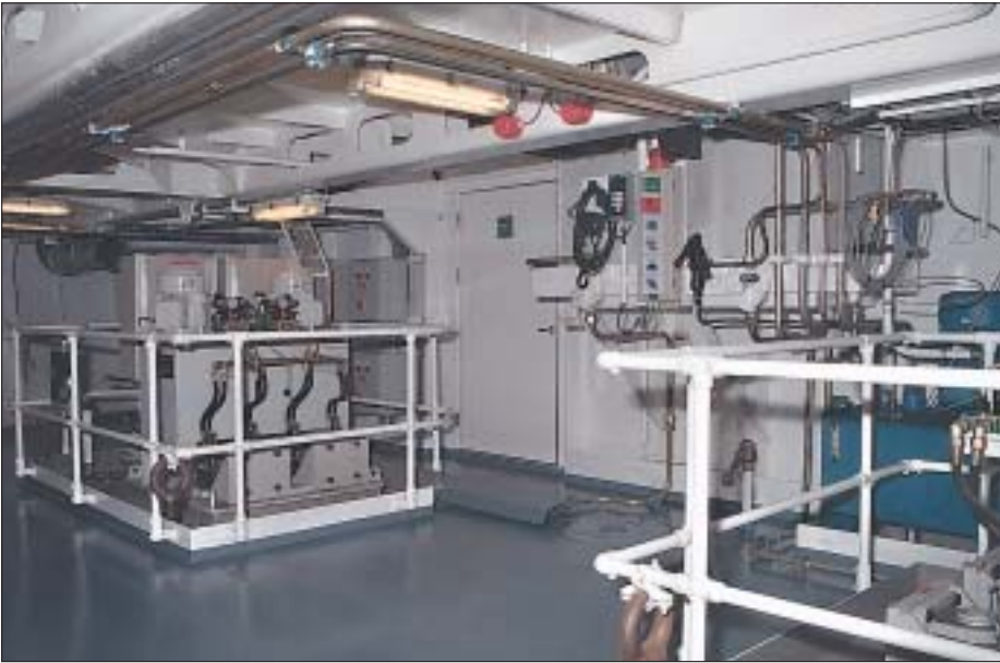
The steering gear comprises two proportional electromagnetic valve groups
