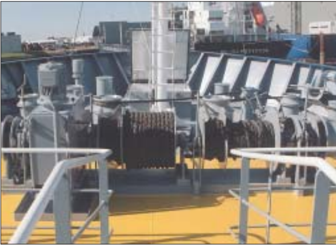
The deckmachinery was delivered by Ship's Equipment Centre
