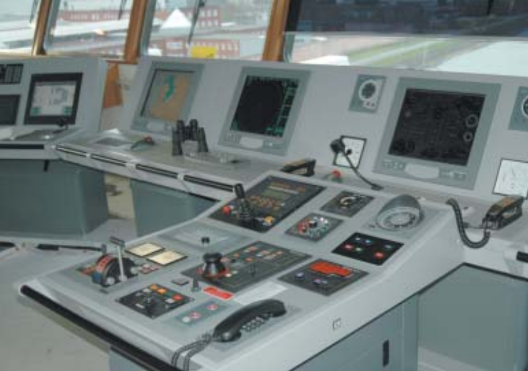
Alphatron Marine Netherlands supplied and installed the navcom installation
