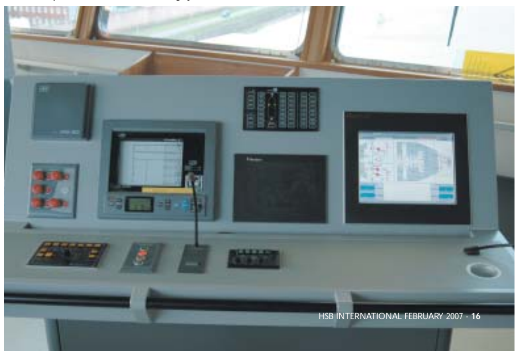
The control panel for alarm- and monitoring systems
