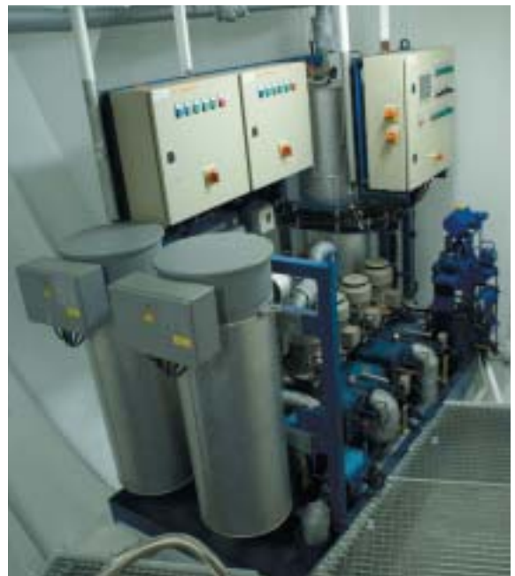
*The booster unit heats the heavy fuel to decrease its viscosity
