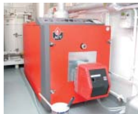
ACV central heating unit
