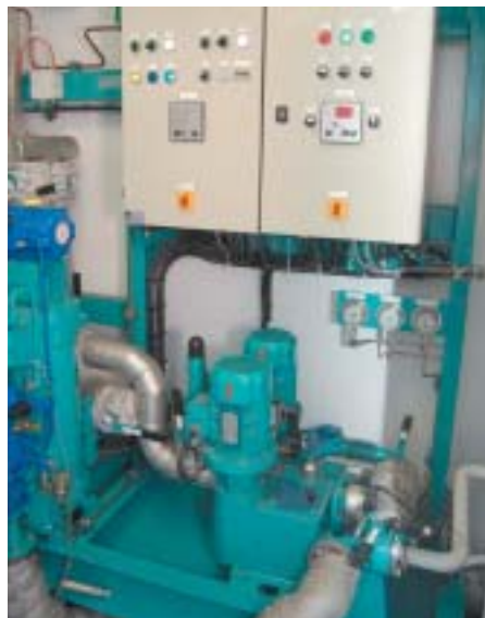
Eefting Engineering HFO booster unit
