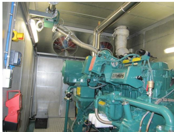
Photos: The new biogas installation is powered by a Perkins 4006-23TRS2 gas engine.
