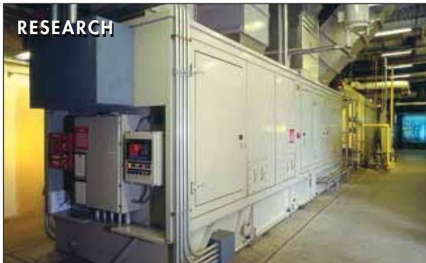
A 5.2 MW *Taurus 60* cogeneration system with on-skid controls serves this pharmaceutical research facility in Wallingford, Connecticut, U.S.A.
