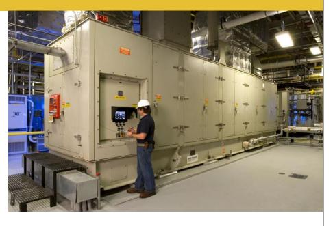
firm was retained to study the project. After careful consideration, a 5.7 MW Taurus™ 60 was chosen as the primary power generation equipment. Coupled with a waste heat recovery boiler, the Taurus 60 gas turbine generator set would provide the campus with both the power and steam it needed.
