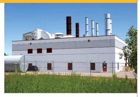
housed in an existing 200,000 square foot warehouse on the property, and a *Centaur*® 40 natural gas turbine, designed and manufactured by Solar Turbines, was the equipment of choice. The gas turbine produces 3.4 MW of electricity and can generate up to 50,000 pounds of steam per hour. The steam provides for all of the medical center's heating needs, and when run through an evaporative chiller, handles most of the warm weather cooling needs.
