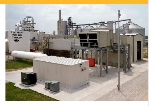
Solar's extended scope of supply included the complete power island, consisting of the gas turbine, unfired heat recovery steam generator, and fuel gas compressor. The *Mars* gas turbine operates 100% base load and is equipped with *SoLoNOx*<sup>™</sup>, Solar's dry low-emissions combustion system, required to meet stringent air emissions regulations.
